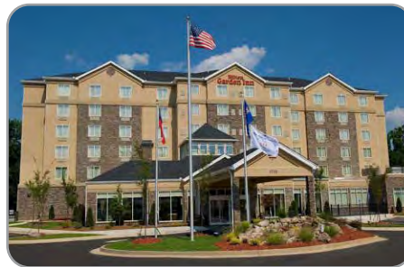
Hilton Garden Inn 1735 Browns Bridge Road 770-532-3396
